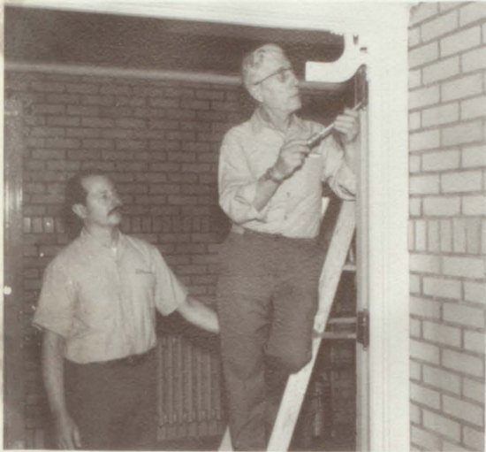
Messrs. Goione and Madonna are busy replacing "door checks."
