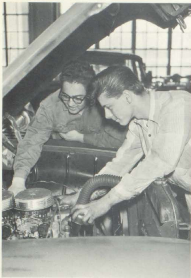
Adjusting Carburetors
